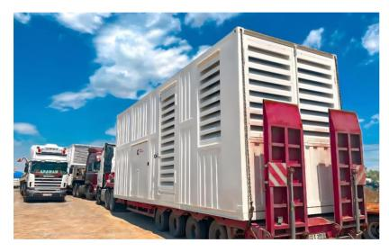
• Supply & installation of perkins generator 400/231v 1500 rpm 50hz
